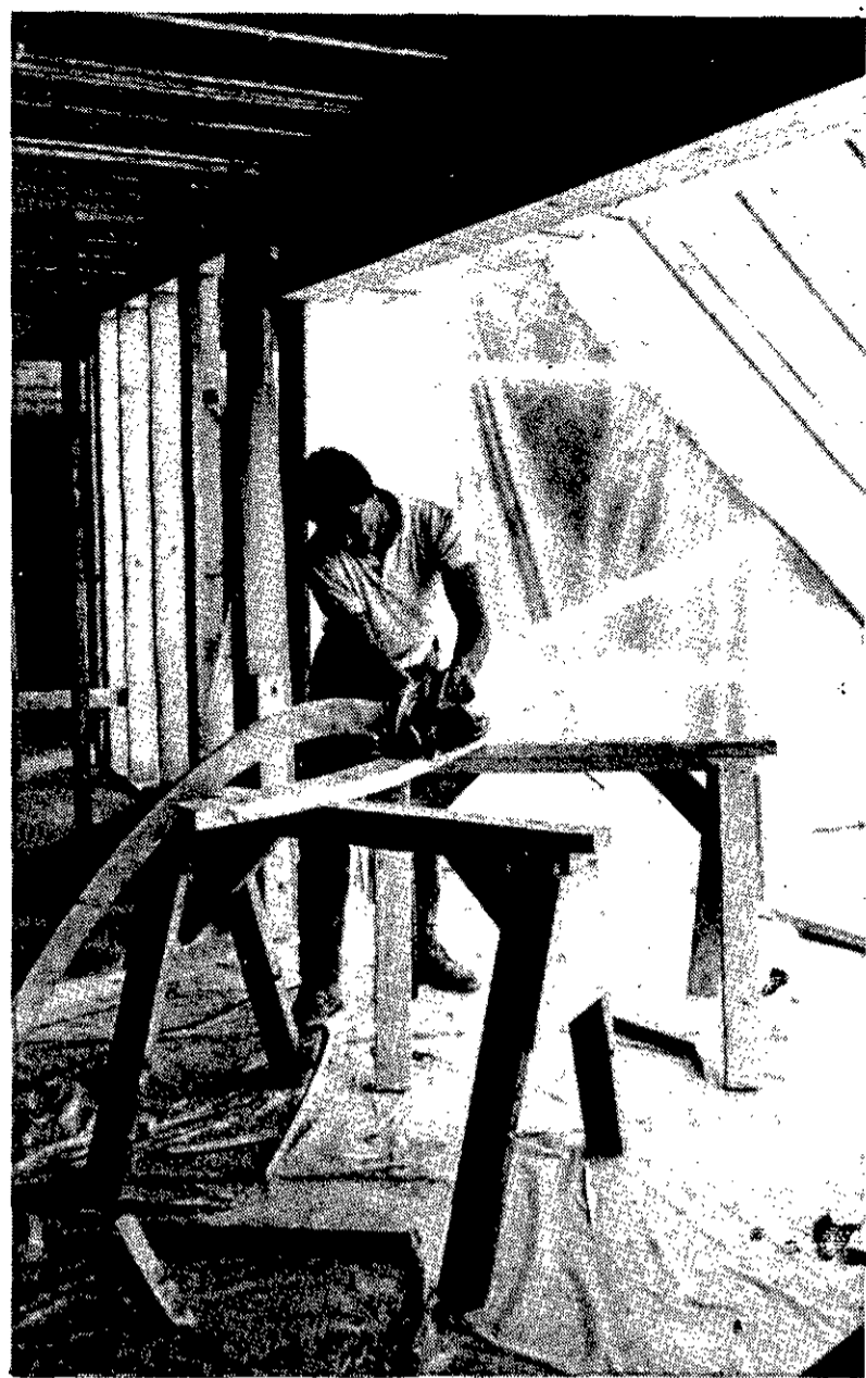
Cutting radiuses for a spiral stair case, construction laborer Bill Senecal uses the natural light provided by the adjacent sun room in this custom Barsons Construction home in Voorheesville. The sun room will be constructed using tempered glass. One of the many extra insulating techniques used in this construction is the use of two inch thick rigid styrofoam on all outside corners. Lorraine C. Smith
