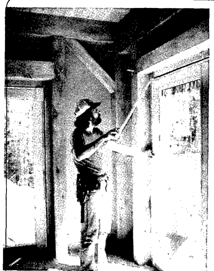
From Kaatskill Post & Beam, Feura Bush, supervisor Mike Pabero measures the picture window for trim. The post and beam structure, shown here, offers aesthetics and long lasting qualities, and also allows the outside walls to be constructed stud free with stress skin panels. This house construction technique offers an uninterrupted envelope of energy efficient insulation with very low infiltration, the builders say. This Voorheesville house will also utilize high-energy trusses to accommodate insulation for a R-value of up to 45.
