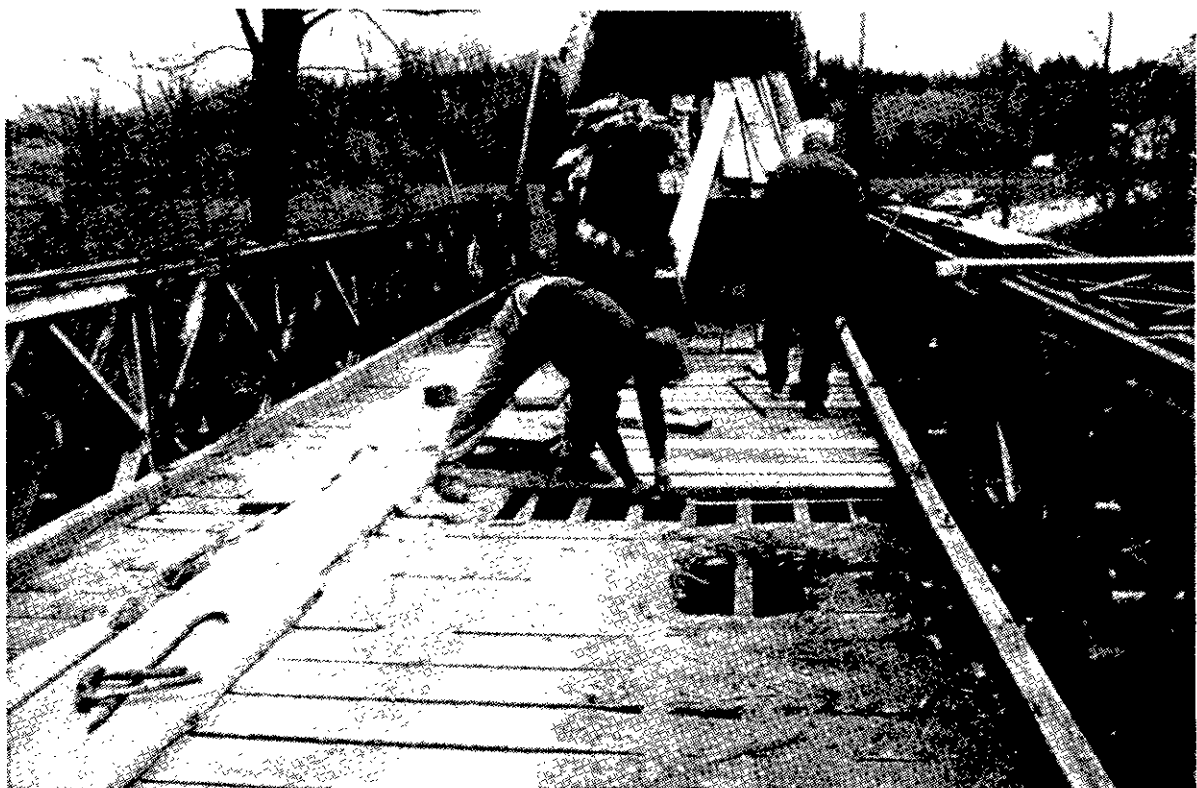
Crews from the Town of New Scotland repair the wooden deck of the Onesquethaw Creek Rd. bridge for normal wear and tear. The bridge is scheduled to be replaced by 1988.
