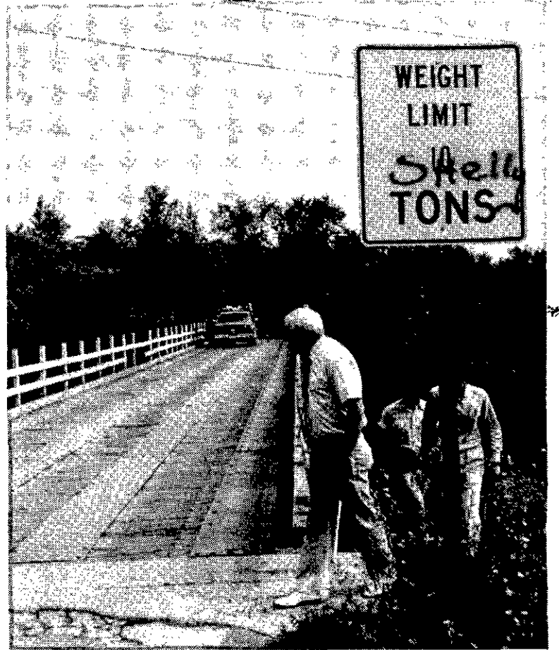
As Bethlehem Supervisor J. Robert Hendrick leads the way back to road level after the inspection, a truck rumbles over the Rockefeller Rd. bridge just hours before it was closed to all traffic Friday. The bridge had a 10-ton weight limit. On the cover: Under the bridge, engineer James Walrath points to a deteriorated joint. Spotlight.
