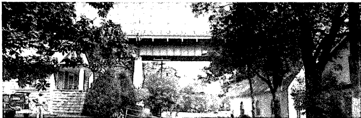
The Delaware Ave. bridge was built in the early 1930's and spans Normansville and the Normanskill, leaving them both in its shadow. The bridge has been given a "two"
