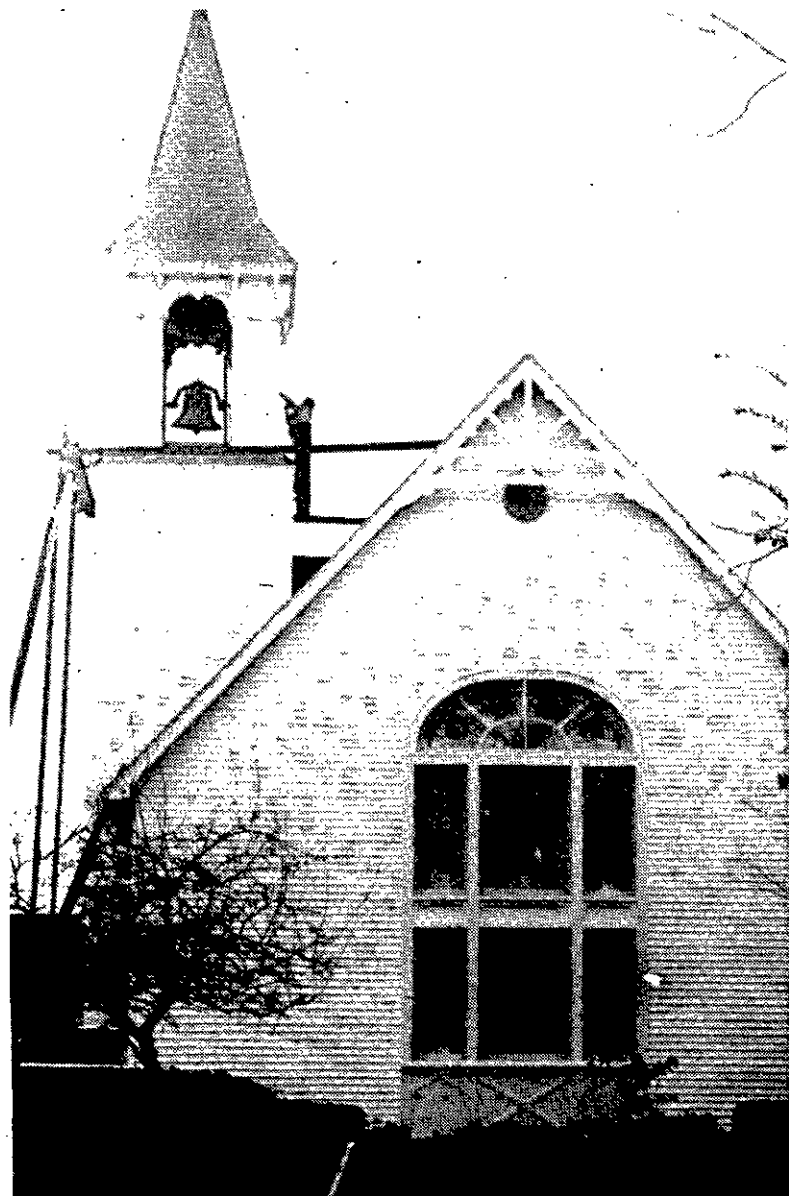
A workman is silhouetted against the sky as he puts siding on the bell tower of the First United Methodist Church of Voorheesville. The church, which has been undergoing renovation, will host the annual "hanging of the greens" Saturday, Dec. 12. Lyn Slapf
