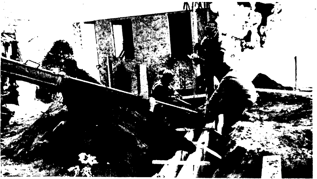
A crew from Northeast Custom Builders pours concrete for a garage addition on Borthwick Avenue, Delmar, using forms from RVG/Thermal wall in Chatham. A new technique in the U.S., foam allows
