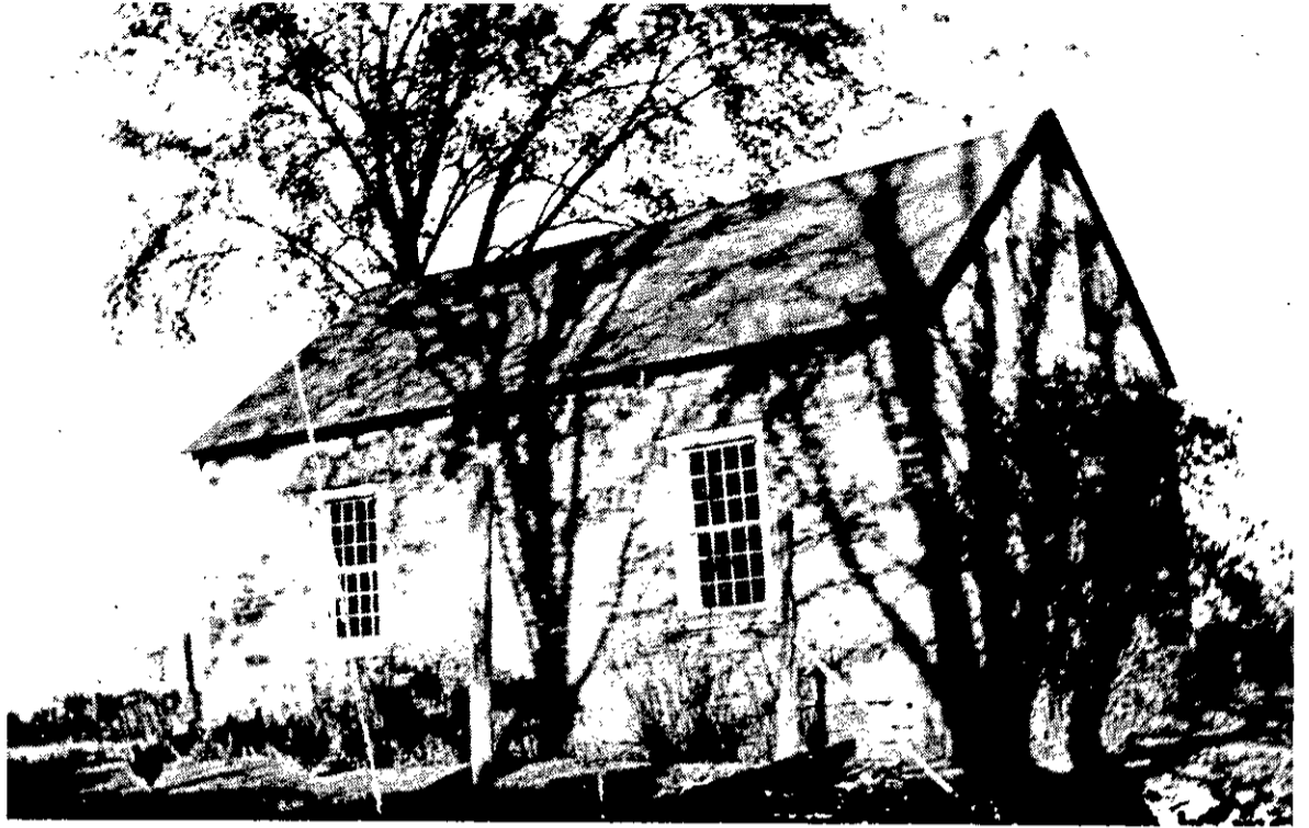
A pre-1940 photograph of the Leonard house shows the Van Dyke Road side of the house. Note the small window in the gable end.
