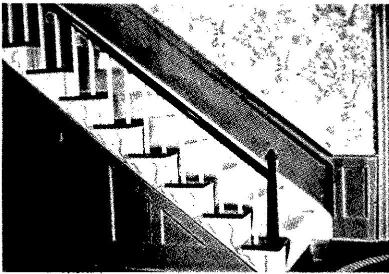
The short banister and low handrails may have been installed on the stairs to give better proportion to the hallway.
