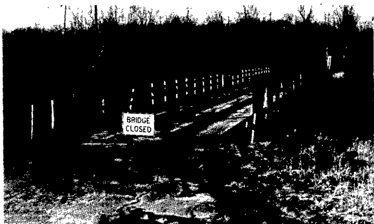
The closed Rockefeller Rd. bridge stands in a worsening state of deterioration and neither the Delaware and Hudson Railroad or the town are in a position to repair or replace the bridge.
