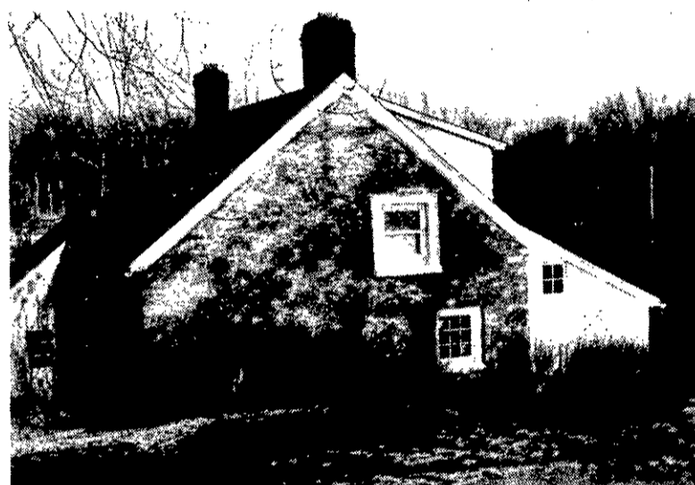
Above, a front view of the 1791 Van Etten house. Below, the house is built into the hill that adjoins it on the west side. Elaine McLain
