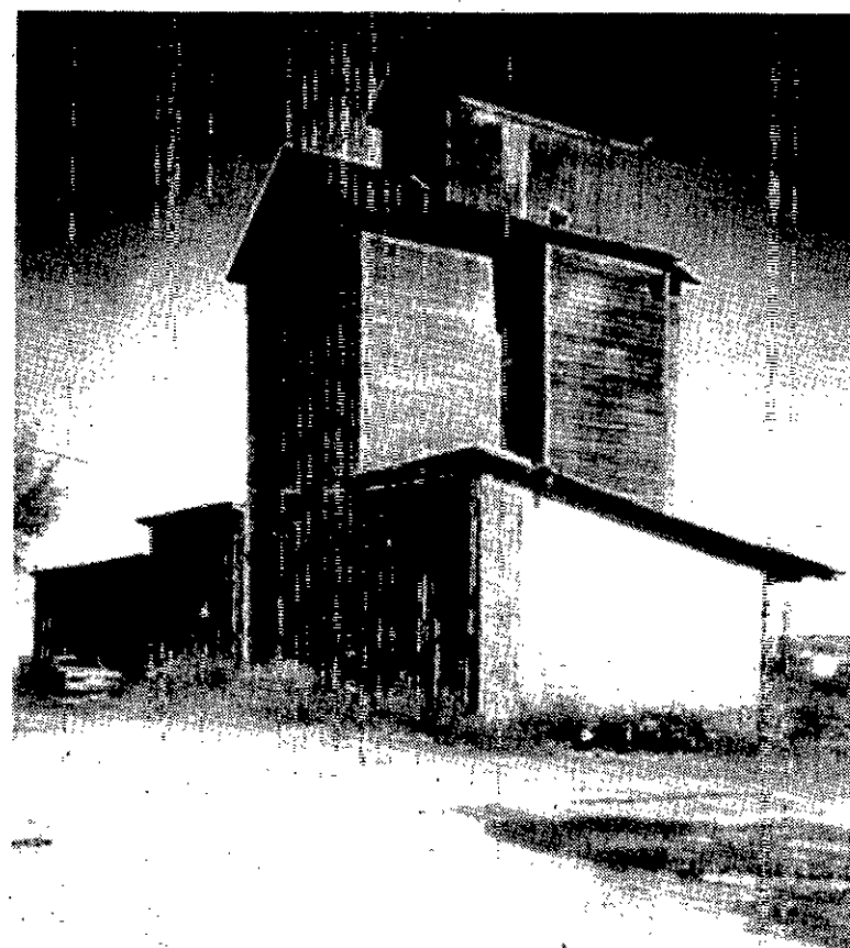
Occupying site of proposed Feura Bush Stewart's shop is this dilapidated grain elevator. Bob Hagyard
