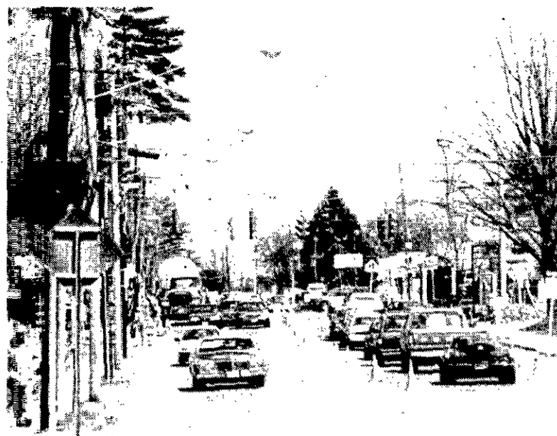
Traffic stacks up on Delaware Avenue as crews begin to install a ramp from Elsmere Avenue. The ramp will allow Elsmere Avenue motorists to turn right onto Delaware without waiting for the stop light.
