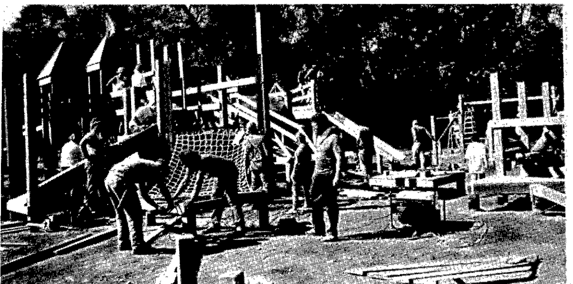
Volunteers from the Bethlehem area gathered recently at South Bethlehem Park to build a playground for the children in the community. The project was headed
