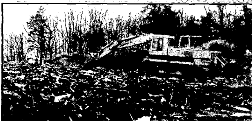
Harlen Metz' Spawns Hollow Road construction and demolition debris landfill. Mike Larabee
