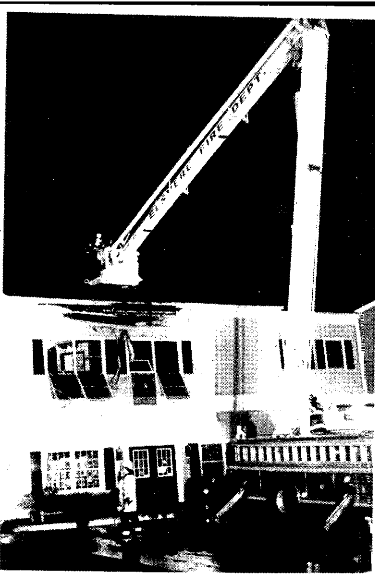
Elsmere Fire Department firefighters go above Mair Square's roof to extinguish Friday night's fire. They eventually cut a hole in the roof for ventilation. Water severely damaged the office of Walden Asset Group and The Toy Maker. Firefighters worked for three hours to put out the one-alarm fire.
