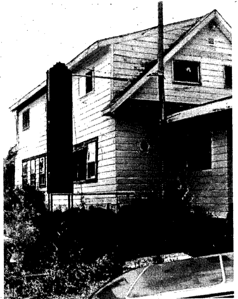
A planned Stewart's store, which won final approval from the Town of New Scotland earlier this month, will replace the dilapidated former Tam Tom Pizza building at the intersection of routes 85 and 443.
