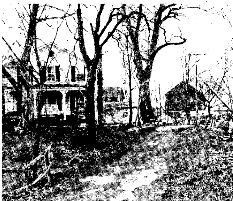
The intervention of a potential buyer, whose name has not been disclosed, could forestall efforts to evict Don Terhune and his children from property adjacent to New Scotland Town Hall for code violations. File photo
