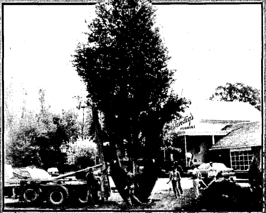
Using the world's largest tree spade, workers from H.E. Jackson of Ballston Lake relocate a 35-foot copper beech away from power lines on the grounds of Verstandig's Florists in Delmar. Dev Tobin
