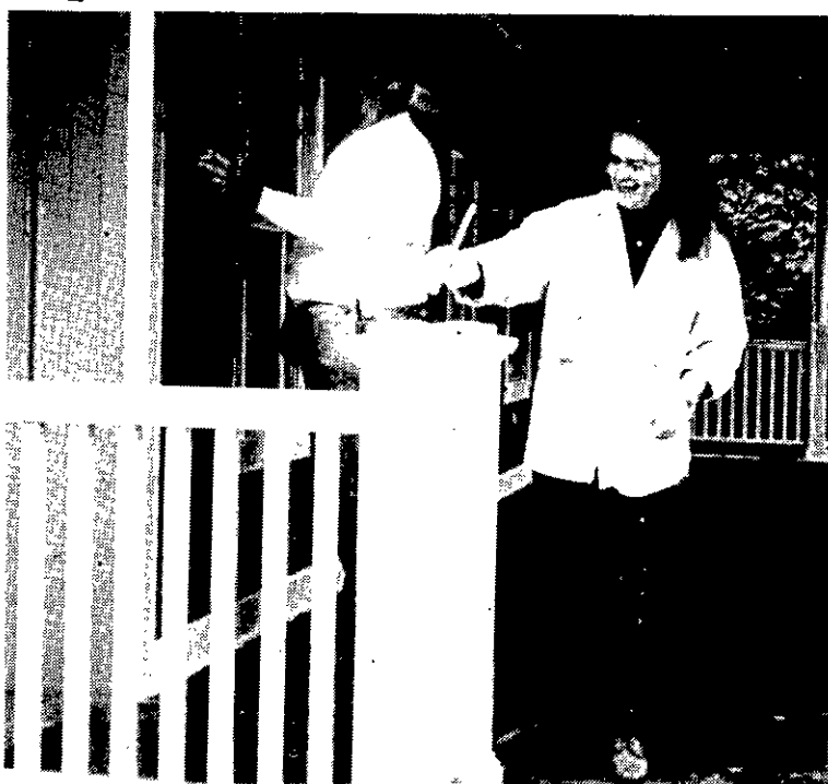
Jim Olsen and store manager Debra MacFarland put the finishing touches on the new addition to the Route 85 business. Dev Tobin
