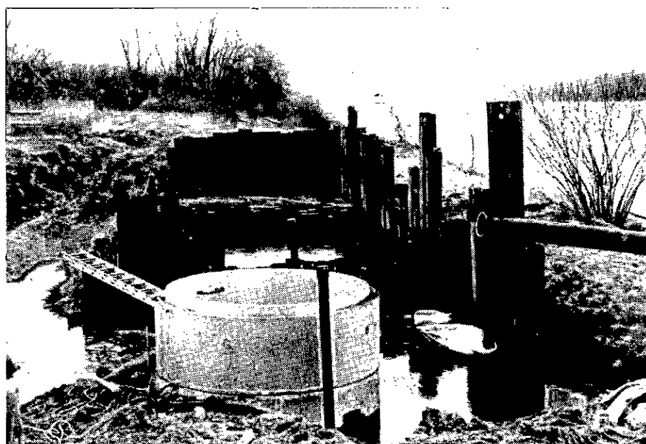
Hudson River Infiltration Gallery under construction
