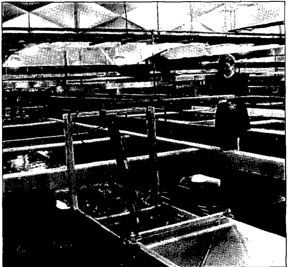
Bethlehem Supervisor Sheila Fuller looks out on the town's new water treatment plant — now in full operation — on Clapper Road. Elaine McLain
