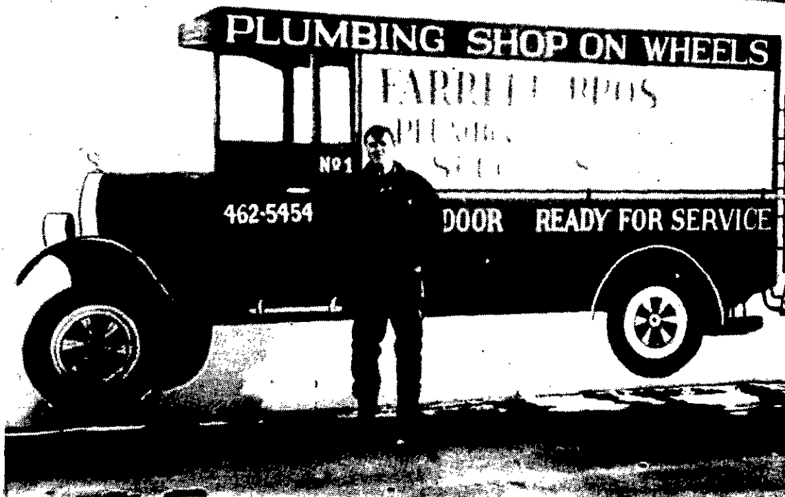
Randy Rowe of Farrell Bros. Plumbing & Heating, Inc. on 300 Delaware Ave. in Albany said his business offers something almost unheard of these days — same day service.
