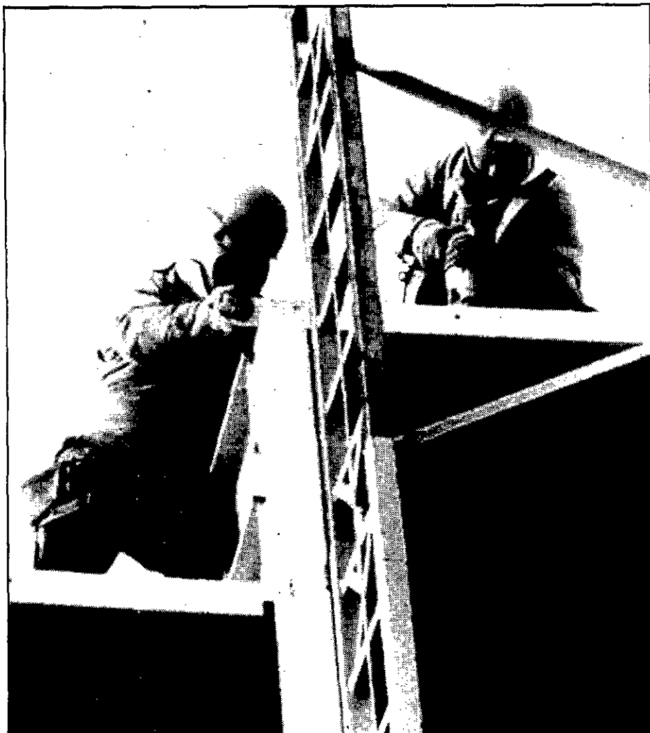
Outdoor construction continues on the new Price Chopper center in Slingerlands despite the sub-zero temperatures that chilled the area this week. Hugh Hewitt
