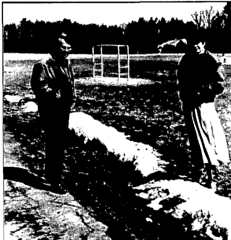
Clarksville Principal Joseph Schaefer and PTA president Melanie Henderson survey the damage caused by poor drainage.
