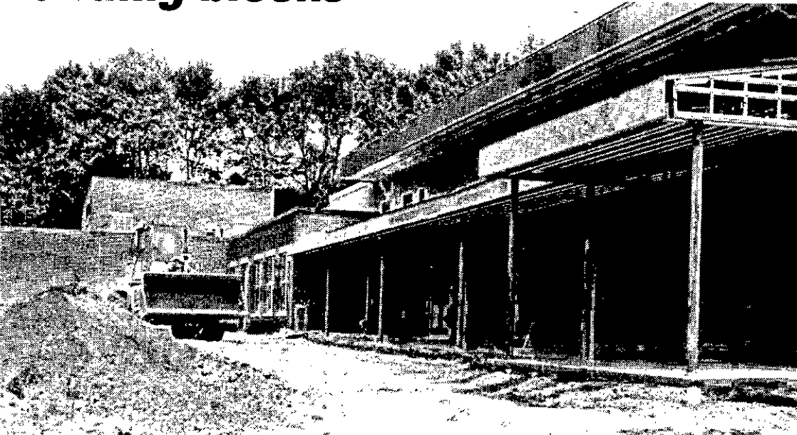
Construction on the Early Learning Center at Slingerlands Elementary School is on schedule. Paul Deys
