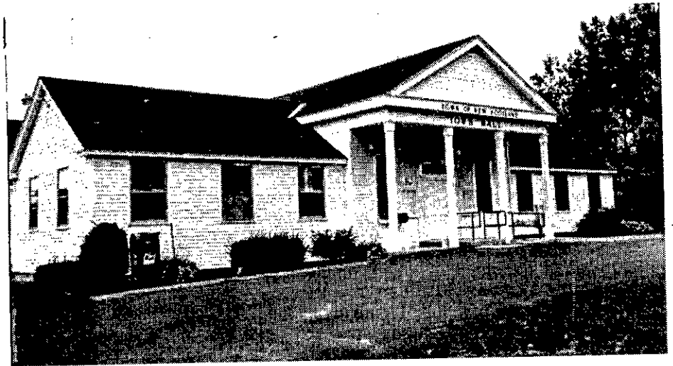
Construction is complete on a $300,000 addition to New Scotland town hall that doubled the building's square footage. Hugh Hewitt
