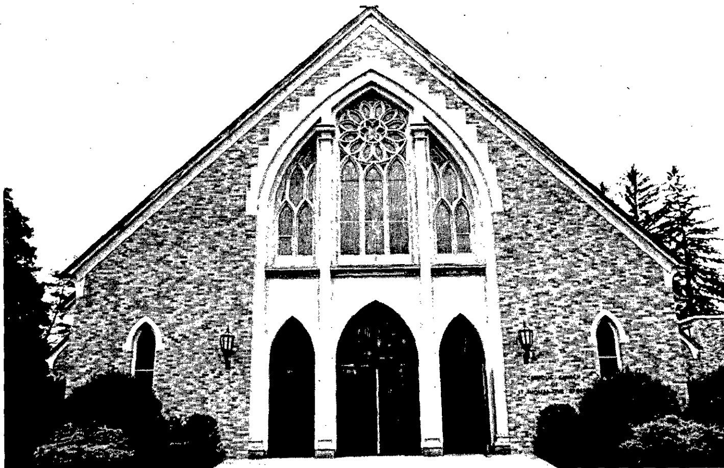
The Church of St. Thomas the Apostle in Delmar is planning renovations for its rectory in a project that involved an addition to the school. Hugh Hewitt
