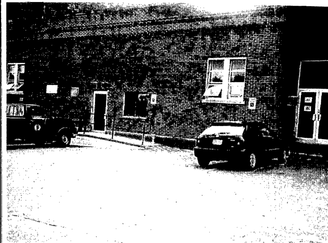
Renovations and plans to move Ravana-Coeymans-Selkirk Community Library to 15 Mountain Road in Ravana are nearly complete. The final move is set for sometime in the middle of October. Until the library completes the move, it is not accepting book donations. To volunteer to help in the move, call 756-2053.
