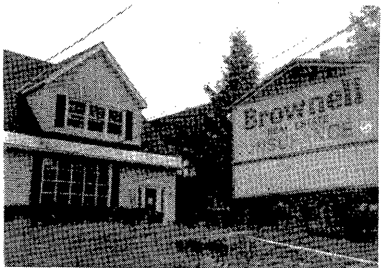
This office building on Delaware Avenue will be demolished to make way for expansion of the Delmar post office's facilities.
