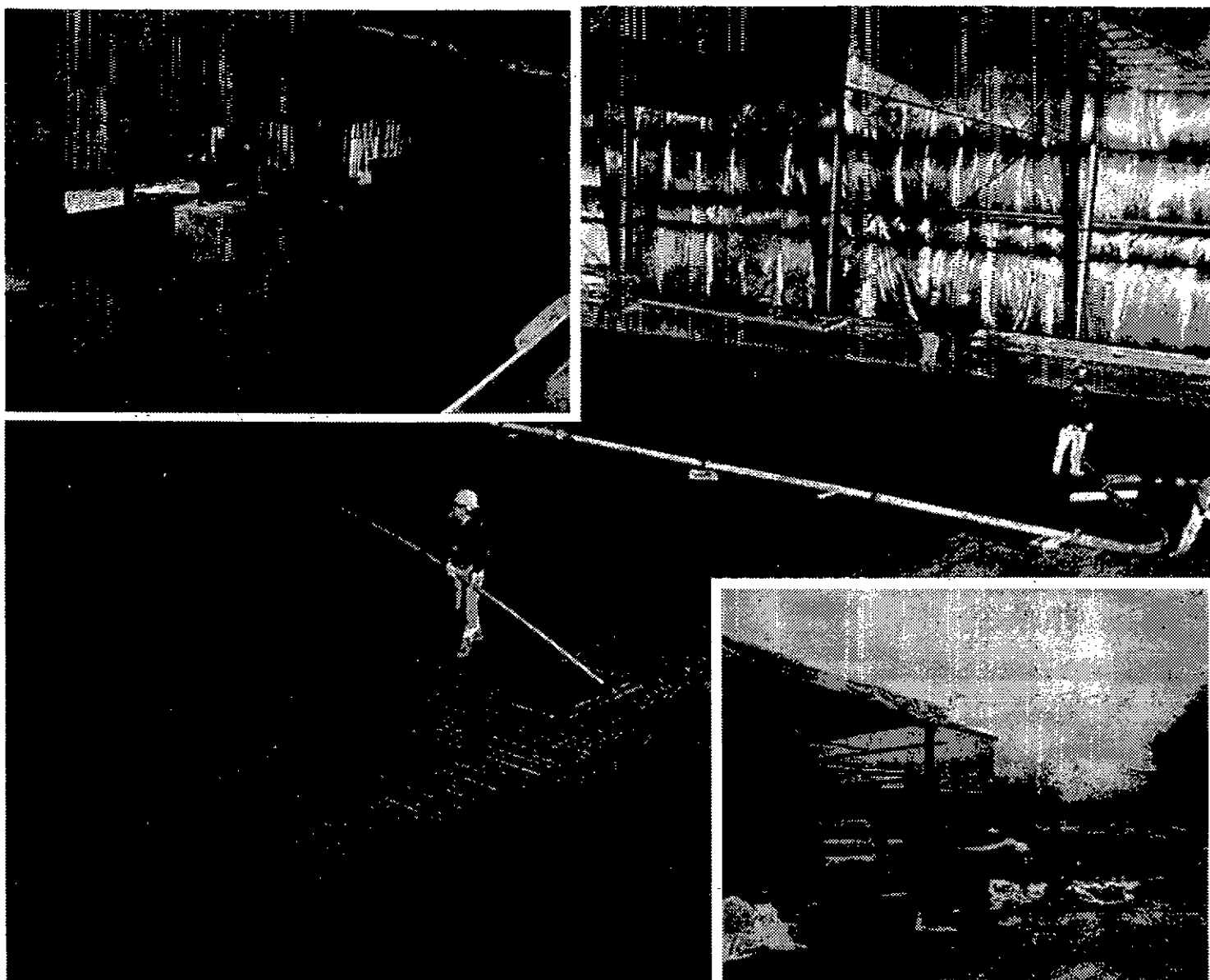
Construction workers pour concrete at the BIG Arena under one of the rinks in the two-rink facility.
