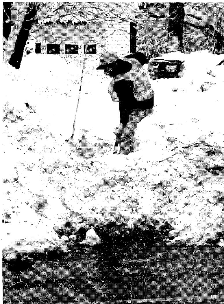
Ross Hendrick, a Bethlehem Highway Department worker shovels snow to clear a hydrant. The town has more than 1,600 fire hydrants — and many are still buried in snow banks. If you can clear snow from a fire hydrant near your home please dig in.
