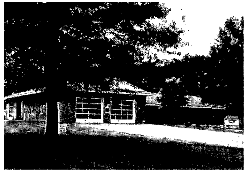
The village of Voorheesville has asked B&L to assist the fire department with addressing the many items that are both deficient and outdated at the 38-year-old firehouse on Route 156 in Voorheesville.
