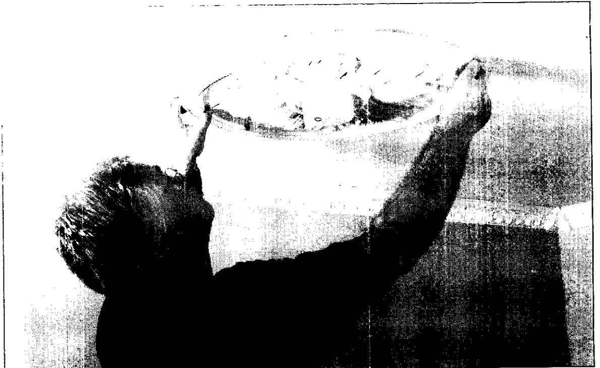
Installing a decorative medallion is easy with the Quick Clips medallion installation system (shown).
