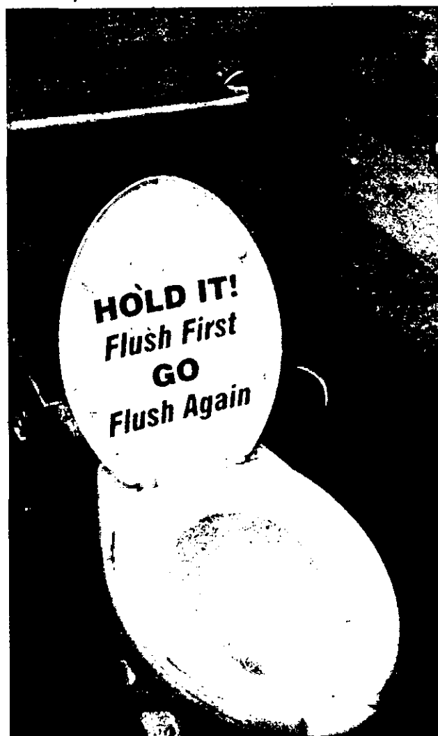
RIGHT: The center's new bathroom facilities use only one third of a cup of water per flush. The toilets operate using mostly gravity to send the waste into a tank beneath the surface of the ground. Once there, the waste is separated into liquids and solids, and the solid waste is left to decompose over the course of five years.
