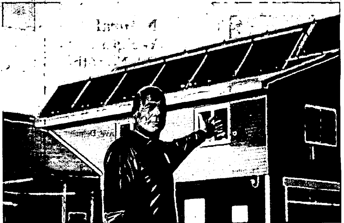
Dennis O'Shaughnessy, owner of Glenmont Car Wash, motions to a bank of 12 solar water heating panels recently installed at his Route 9W business. He hopes the technology will decrease his natural gas bill and carbon footprint while providing his customers with an abundance of hot water all winter.
