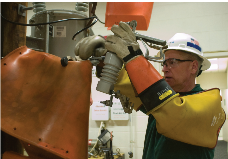
National Grid chief line mechanic Mike Pommer demonstrates how he replaces porcelain insulators during a Nov. 19 press conference. The utility company is busy replacing antiquated equipment before winter begins. John Purcell/Spotlight
