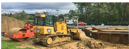
Construction is now underway.
