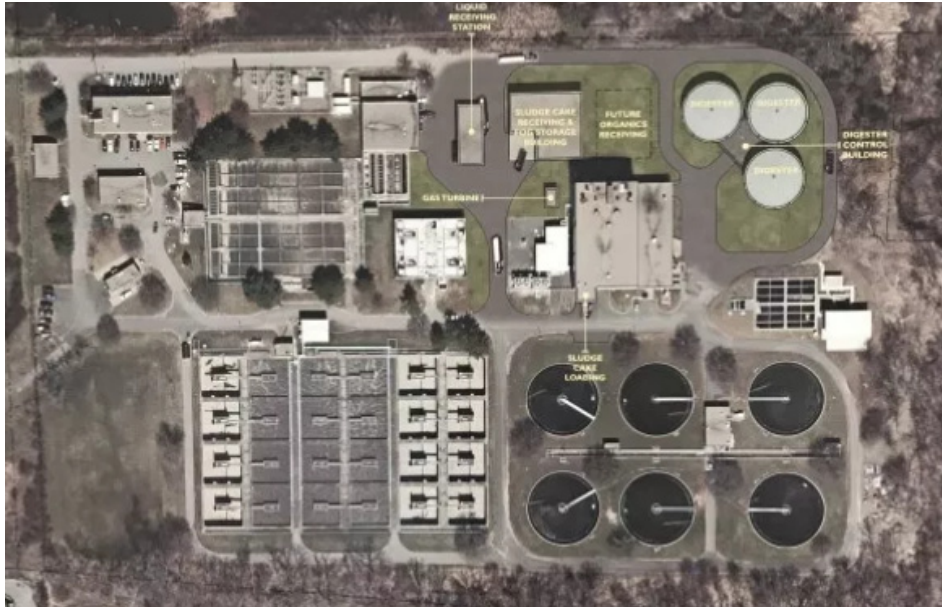
An aerial view of the site that will be transformed into the Albany Saratoga Regional Anaerobic Digester Facility in Menands.
