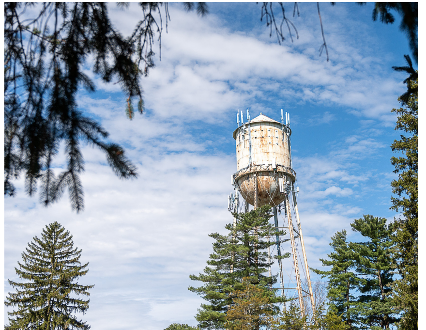
The empty water tower at Kenwood Ave.
